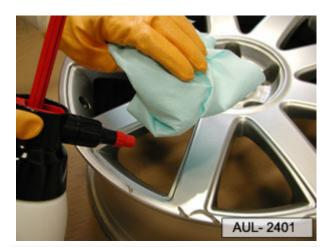
After referring to the maximum deviation sample catalogue to ensure that treatment is permissible, clean the rim with silicone remover
